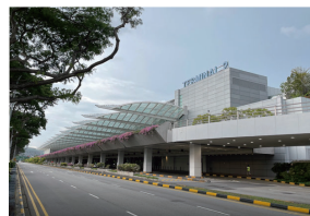
Changi Airport T2 LT REPLACEMENT (2022年竣工)
